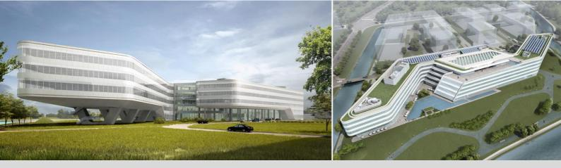
Designed by global architectural firm Gensler, the Shanghai headquarters of Johnson Controls is a fivestory campus with an automatic internal shading system and insulation technologies to manage indoor temperatures, a rainwater harvesting system covering 50% of the building's green rooftop, and a solar hot water system, among other sustainable design features.
