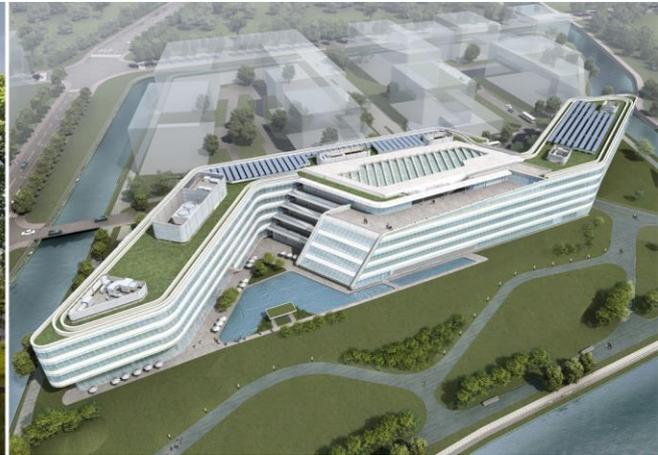
Designed by global architectural firm Gensler, the Shanghai headquarters of Johnson Controls is a five-story campus with an automatic internal shading system and insulation technologies to manage indoor temperatures, a rainwater harvesting system covering 50% of the building's green rooftop, and a solar hot water system, among other sustainable design features.
